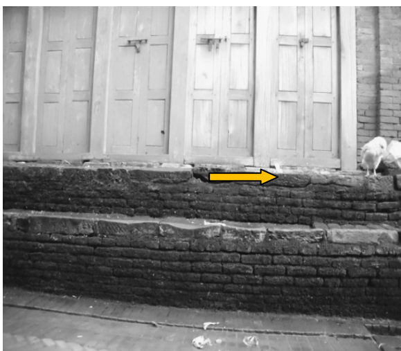
Fig 3 The plinth provided in a building
