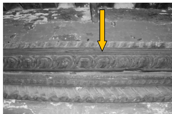
Fig 6 Wooden lintel band
